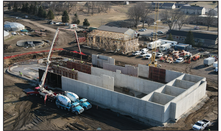
Progress at the wastewater treatment facility has continued through the winter. The construction of a new tank (above) and the expanded oxidation ditch (right) are still underway.
