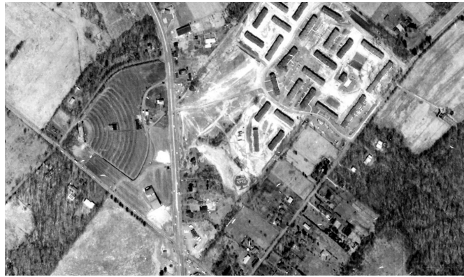
Circa 1970s aerial of the intersection of Welsh Road and Route 309 showing the English Village Apartments under construction.
