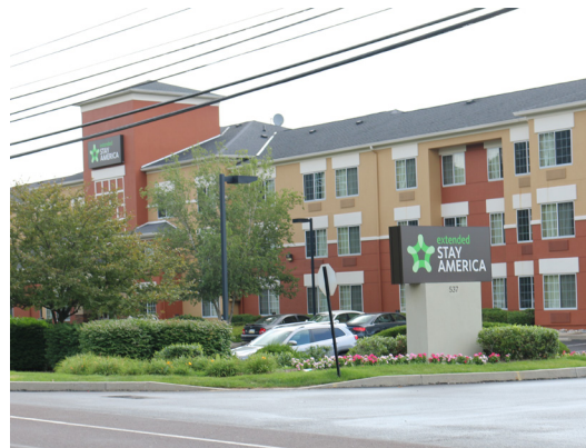
The 136-room Extended Stay America hotel was built on Dresher Road in 1998.
