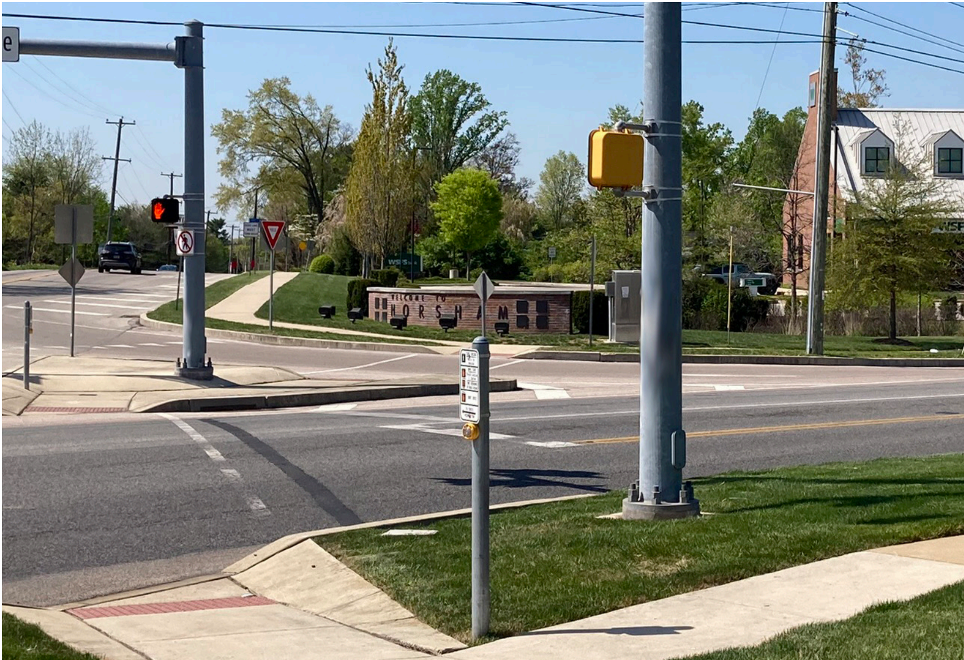
Recent intersection improvements at Welsh Road and Limekiln Pike expanded the sidewalk network, improved pedestrian crossings, and added dedicated turn lanes for vehicular traffic flow.
