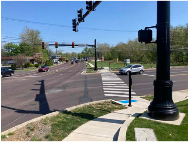
Many of the township's signalized intersections have been upgraded with continental-style crosswalks, ADA curb ramps, and pedestrian push-button signals.
