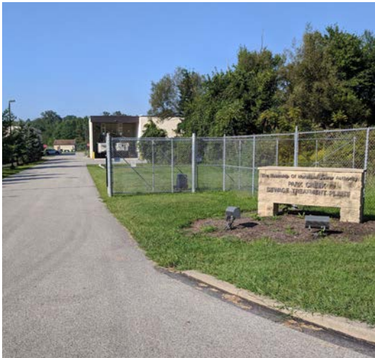
The HWSA's Park Creek Sewage Treatment Plant is located off of Keith Valley Road.
