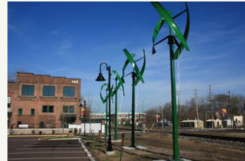
Example of small-scale vertical axis wind turbines installed in the parking lot of the Montgomery County Community College campus in Pottstown Borough.
