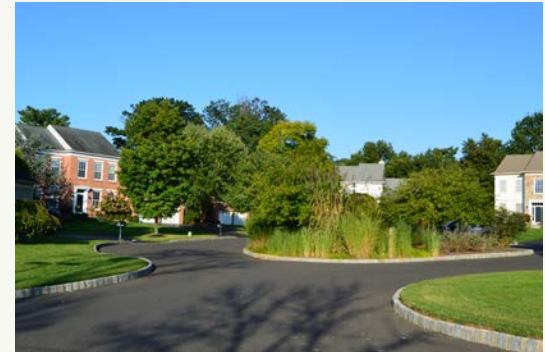
Landscaped cul-de-sac islands, such as this one in the Talamore at Oak Terrace subdivision, can help mitigate the effects of adding the impervious surfaces associated with development, while also improving the aesthetics of a neighborhood.
