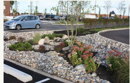
The parking lot islands at the Horsham Gate Shopping Center incorporate attractively landscaped biofiltration basins to capture and infiltrate stormwater runoff from the adjacent parking lot.
