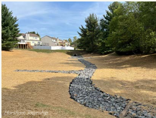
Naturalized stormwater basins, such as this one in Cedar Hill Road Park, are designed to provide greater water quality and habitat benefits relative to standard detention basins.
