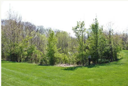
Naturalized stormwater basins, such as this one in Cedar Hill Road Park, are designed to provide greater water quality and habitat benefits relative to standard detention basins.
