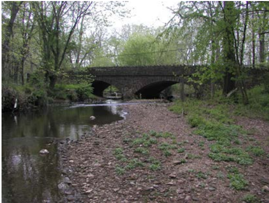
Historic Keith Valley Road bridge over Park Creek.
