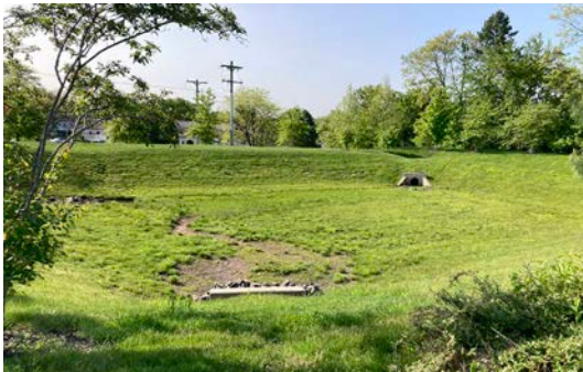
A large stormwater basin was added to the site as part of the most recent improvements.
