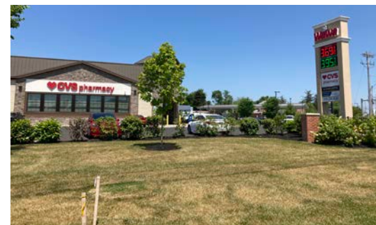
This multi-use redevelopment reconfigured the intersection of Easton Road and Blair Mill Road from a 5-point intersection to a more standard, 4-point intersection.
