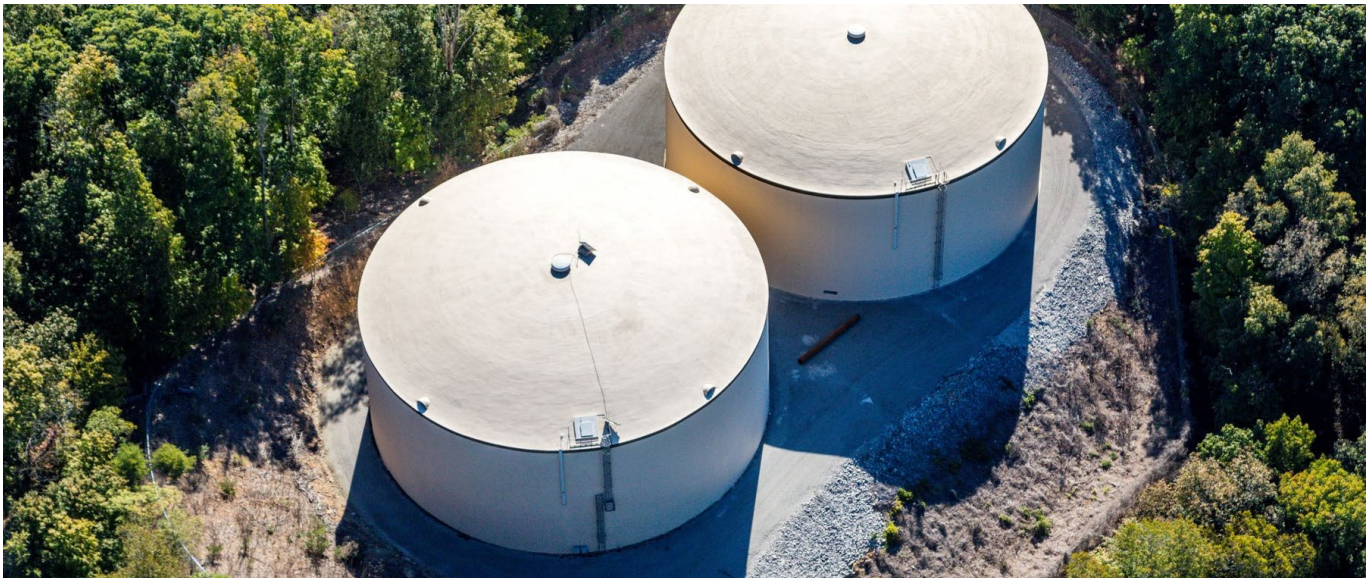
Twin 5 Million Gallon Water storage facilities and related infrastructure support reliable service for MVUD customers.
