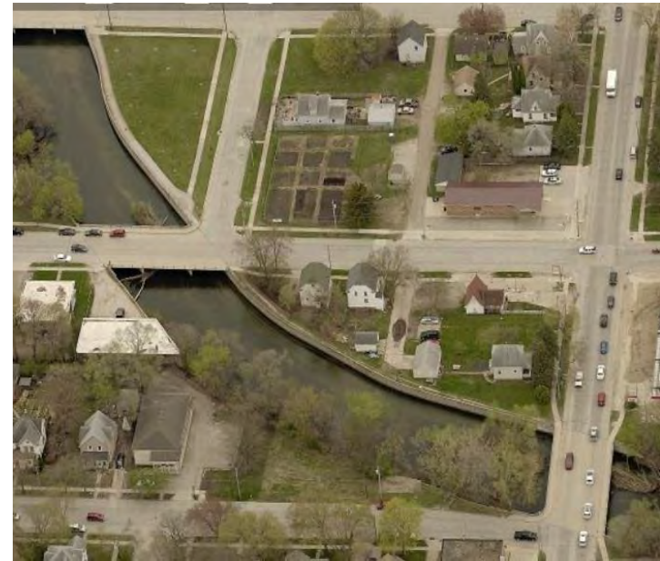
Concrete floodwall on the south side of Willow Creek, between the South Monroe Avenue and 2nd Street SW bridges
