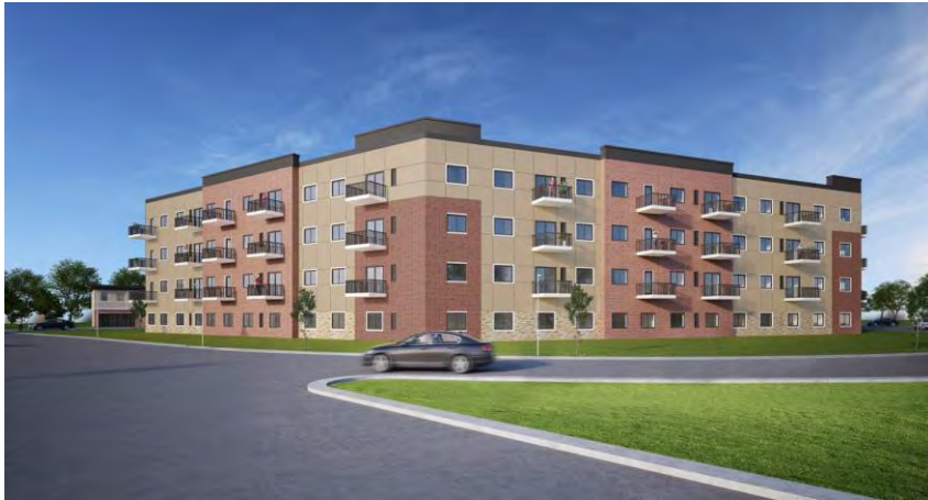
"The River" Apartments, under construction on the former south mall parking lot
