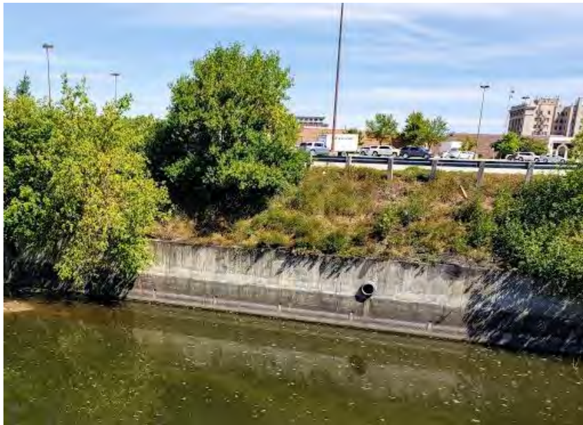
Storm sewer draining the Mall parking lot directly into Willow Creek
