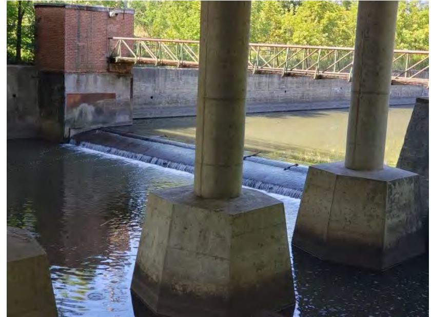
Former Interstate Power dam beneath the South Delaware Avenue Bridge
