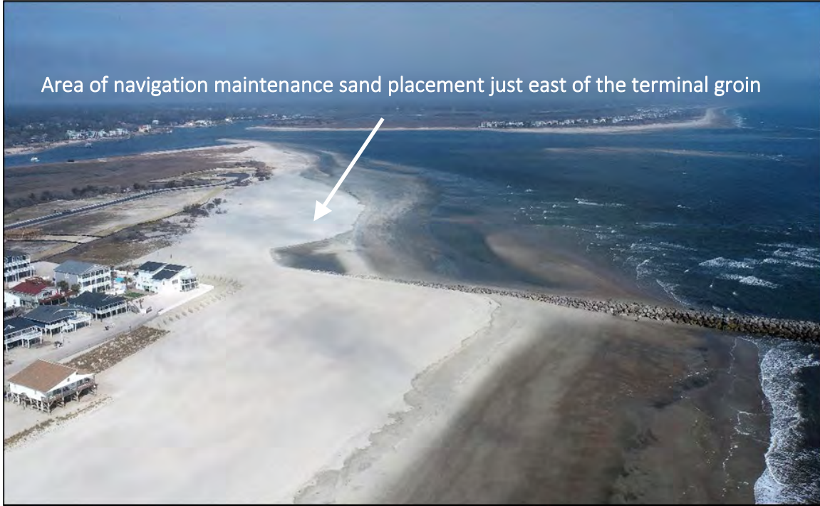
Figure 9. USACE Navigation maintenance material placed east of the terminal groin along the inlet shoreline (Photo taken 2/22/23)
